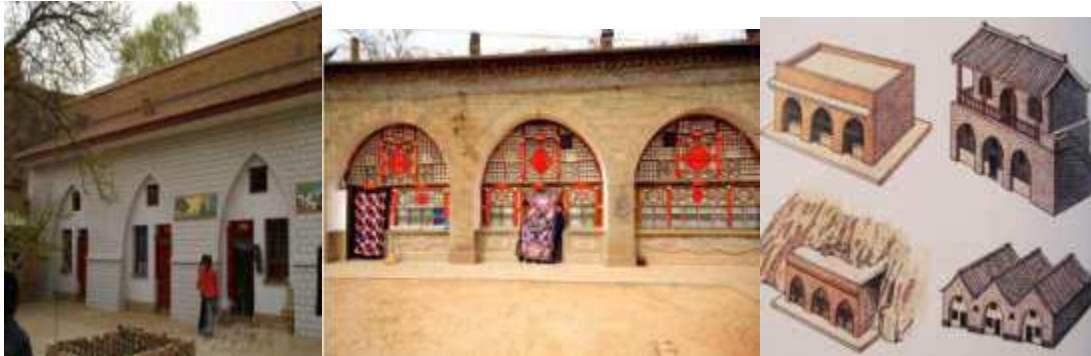
Pic. 3. Furnace circle
